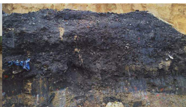
Photograph 4: Preliminary check of heavily contaminated, excavated soils.
