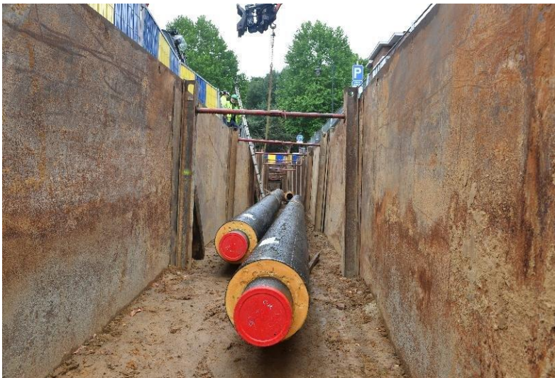
DH Trenches in NOH under construction
