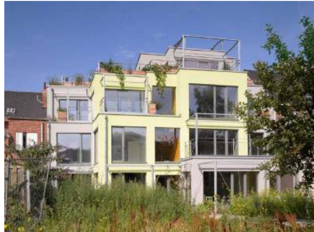
Project Biplan (Batex 55), Architecten : Bxleco1 / FHW © Yvan Glavie
