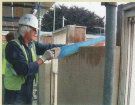
Existing mortar is cut to release stone without causing damage to face edges
