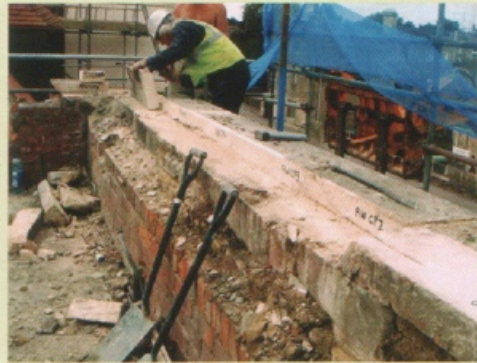
Numbering of stones before removal
