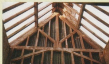
Internal Woodwork Prior to Removal
