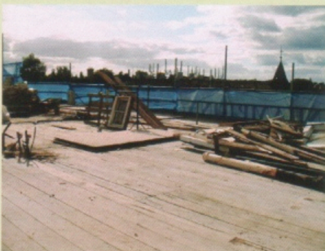
Floorboards to be lifted, August 2006
