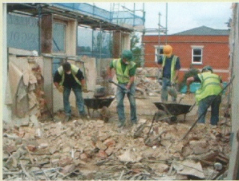
Reclaimed materials: brick, joists, floorboards, precious metals (copper, lead), other metals, internal doors, door hardware, woodwork, general fittings
