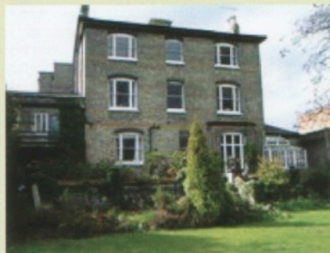
Putney house prior to demolition
