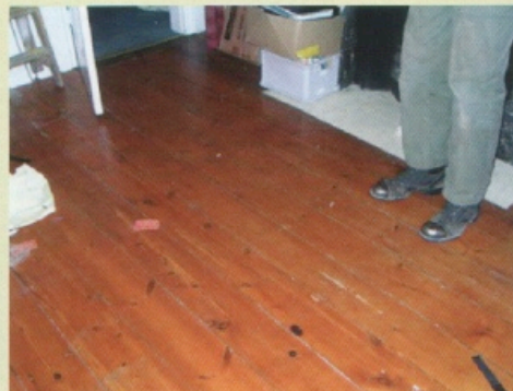
Timber floorboards found throughout the property
