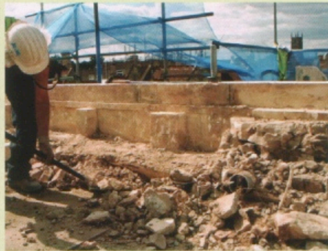
Clearing rubble to expose face stone
