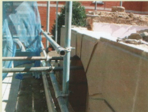
Left front door – scaffold poles used to support stone during dismantle
