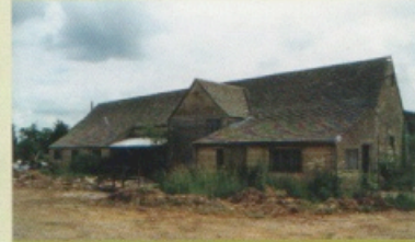
Old Forge Prior to Deconstruction
