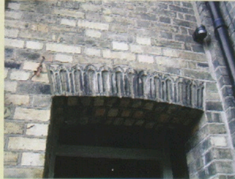
230 tonnes of bricks reclaimed from the houses
