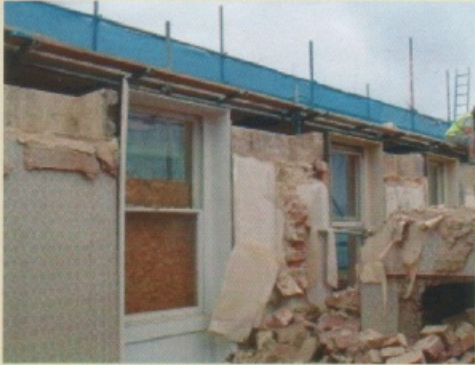
Careful dismantle of window cases to be used in the future
