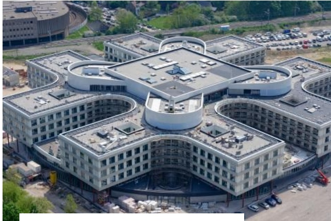
Hôpital Chirec Delta Closed-loop 176 GHE – Depth 90 m
