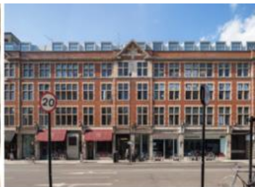
Refurbishment & Fit-out Homes & Commercial Buildings
