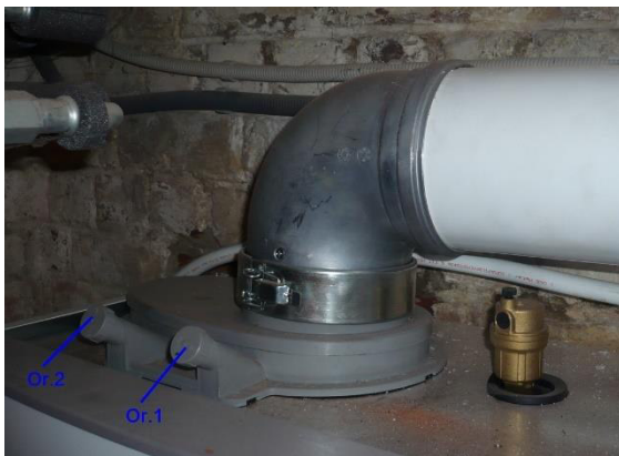
Figure 2 Accessoire comportant 2 orifices de mesure
