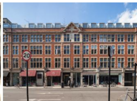
Refurbishment & Fit-out Homes & Commercial Buildings
