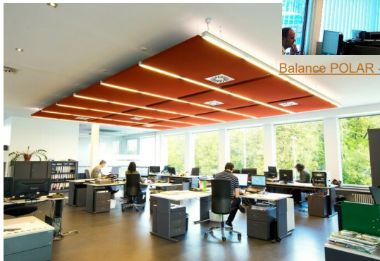
Stereo - Baffles and Ceiling Islands (doxacoustics.eu)
