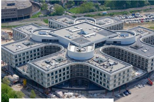
Hôpital Chirec Delta Closed-loop 176 GHE – Depth 90 m
