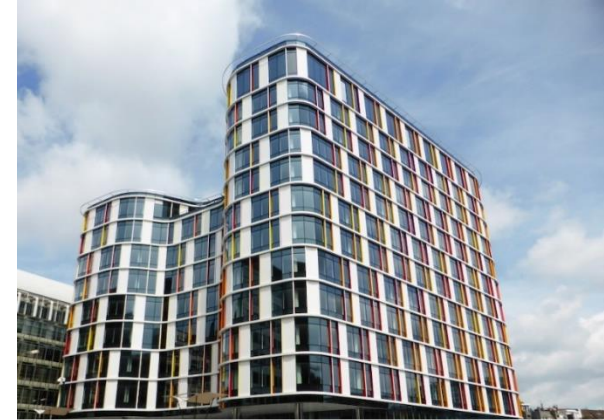
Bât Wilfried Martens Rue Belliard Closed-loop 33 GHE – Depth 240 m
