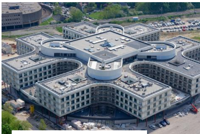
Hôpital Chirec Delta Closed-loop 176 GHE – Depth 90 m
